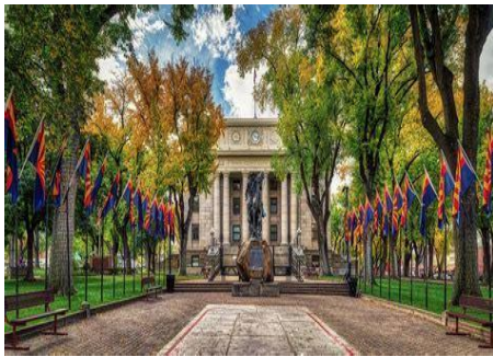
Yavapai County Courthouse
